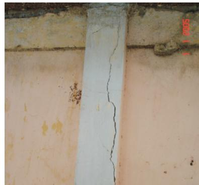
Figure 1. Effect of corrosion of reinforcement in longitudinal cracking in column.
