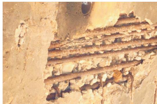
Figure 2. Spalled concrete and reinforcement corrosion
