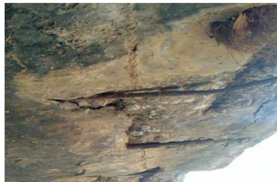
Figure 1. Spalled concrete at the edges
