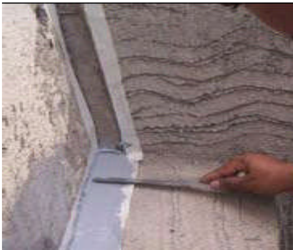
Fig: 4 Tooling of excess sealant
