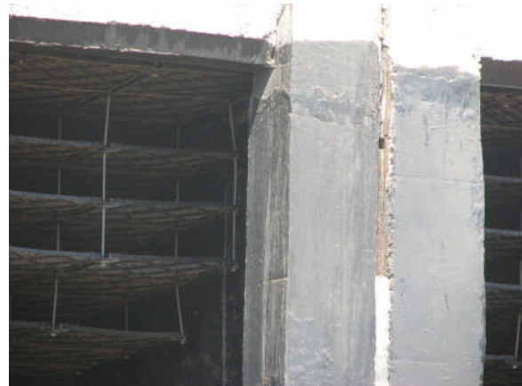
Fig: 2 PU sealant at construction joint
