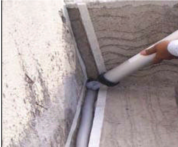
Fig: 3 Application of PU sealant
