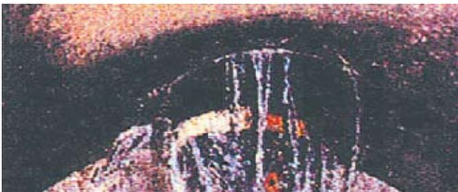
Water enters the manhole due to a pipe penetration.
