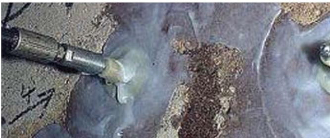
Epoxy injection for repair of crack
