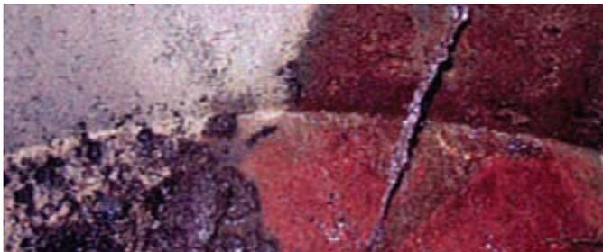
A crack at the base of a manhole allows water to infiltrate.
