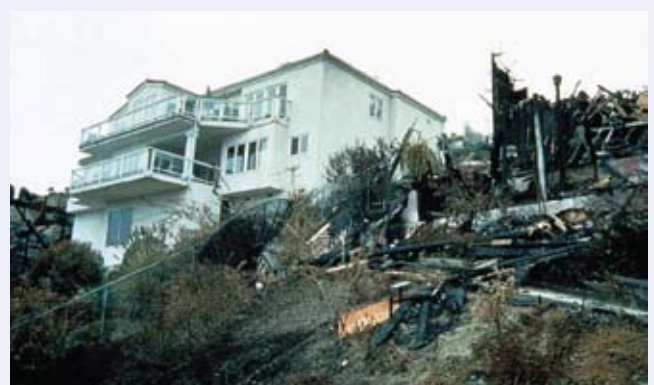
Fig 2: Survival of a Concrete Home in a fire
