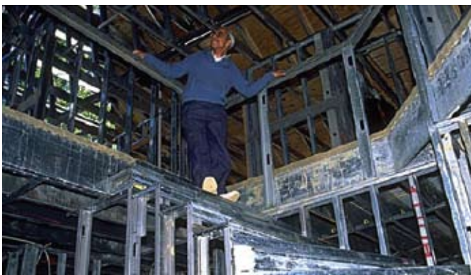
Fig 3: Staircase of composite steel and concrete
