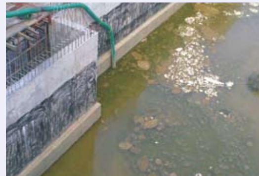
Fig. 3: De-watering by pumping
