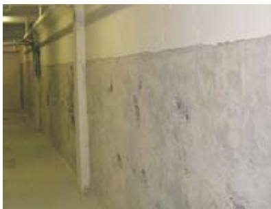
Fig. 1: Surface prepared for application of crystalline coating
