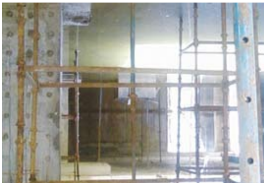
Fig. 4: Basement wall after PU injection
