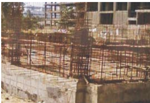
Fig. 2: Raft for structural strengthening
