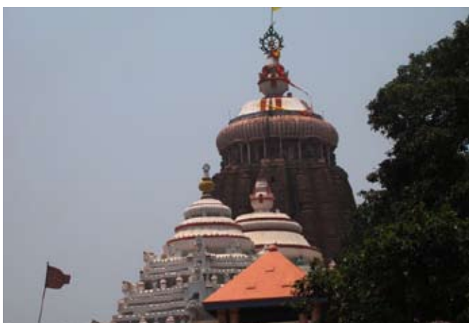
Fig 4: Temple after renovation
