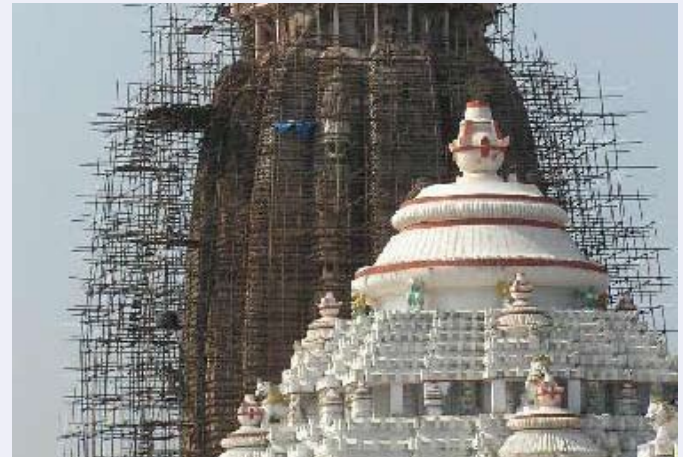
Fig: 2 Renovation of outer face
