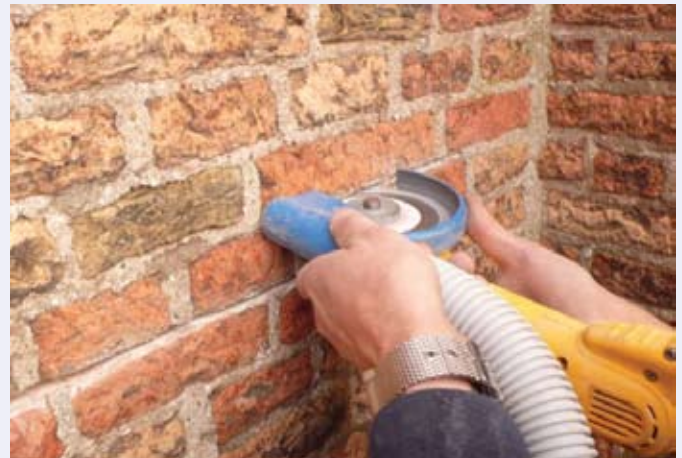
Fig: 6 Raking out of joints mechanically
