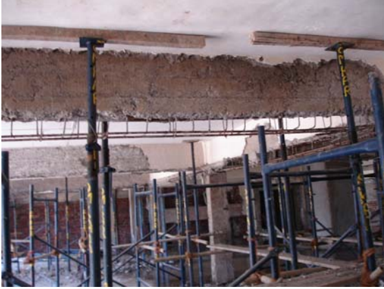
Preparation for micro concrete of a beam
