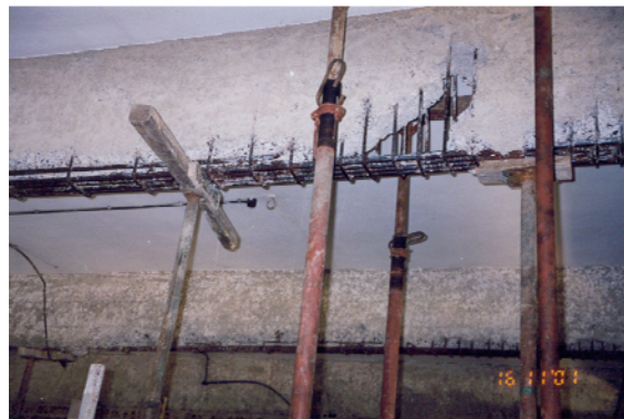
Micro concrete for strengthening of a beam
