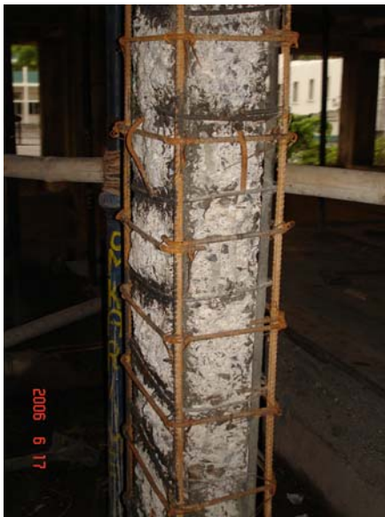
Additional reinforcements provided for jacketing
