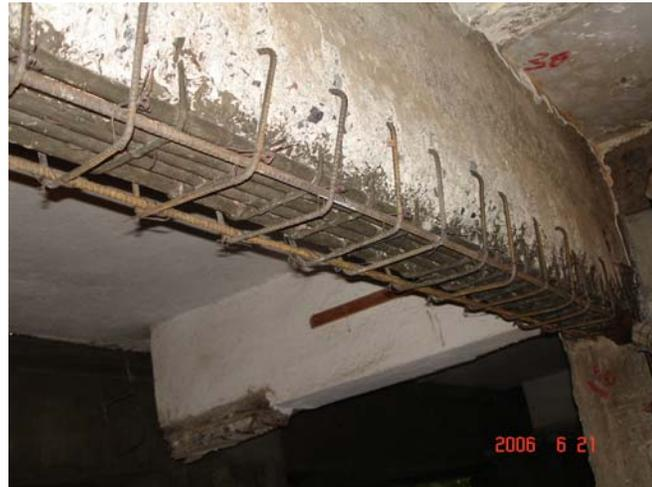
Additional reinforcements and shear connectors provided
