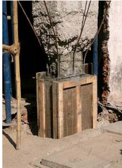
Repair of a column with micro concrete
