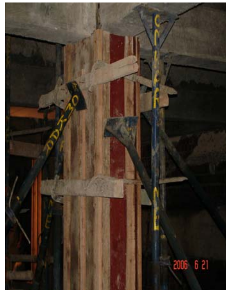
Strengthening of column with micro concrete
