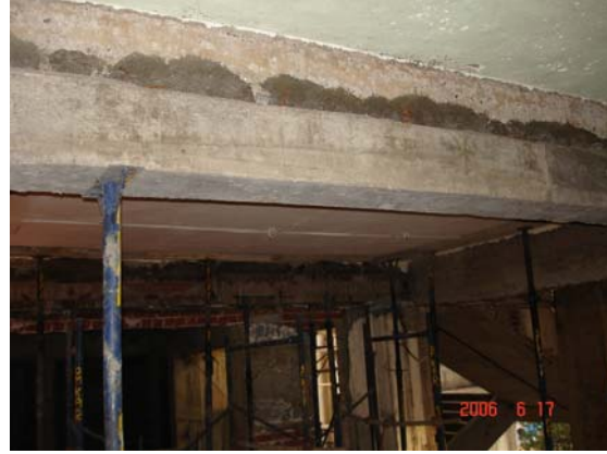
Repair of a beam with micro concrete
