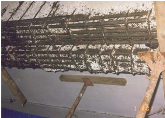
Micro concrete for repair of a congested beam
