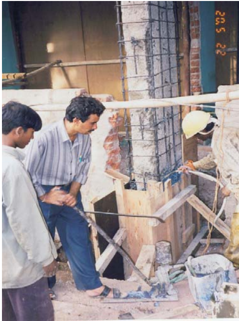
Preparation for micro concrete of a column
