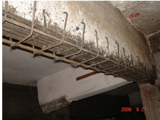
Additional reinforcements and shear connectors provided
