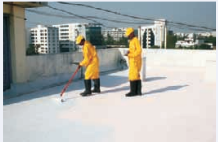
Application of coating with roller - Final coat
