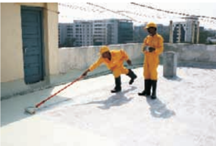
Application of coating with roller - 1 st coat
