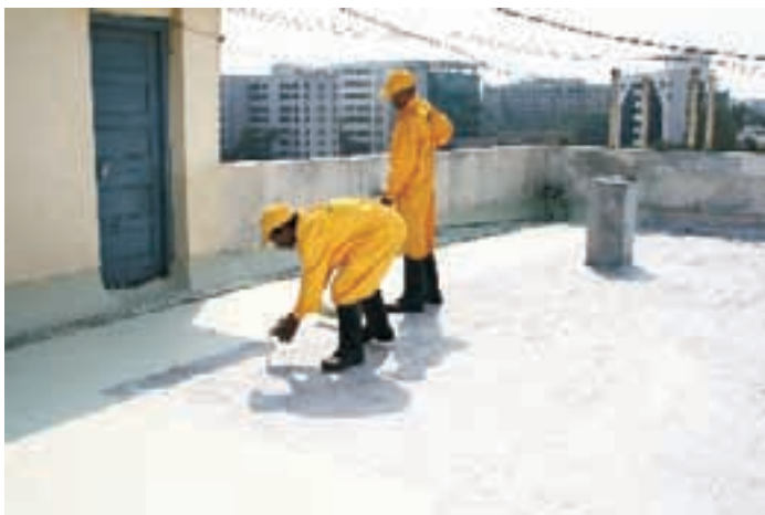
Spreading of material in pre-marked bays
