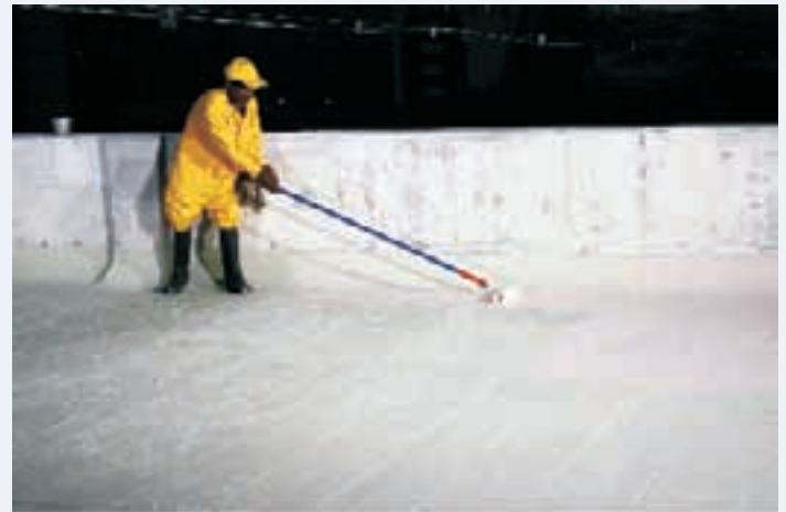
Application of coating with roller - 2 nd coat
