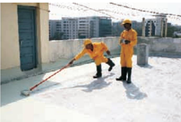
Application of coating with roller - 1 st coat
