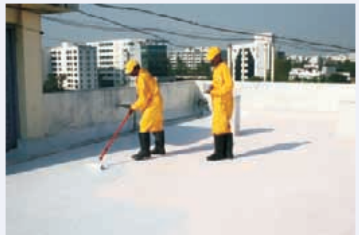
Application of coating with roller - Final coat
