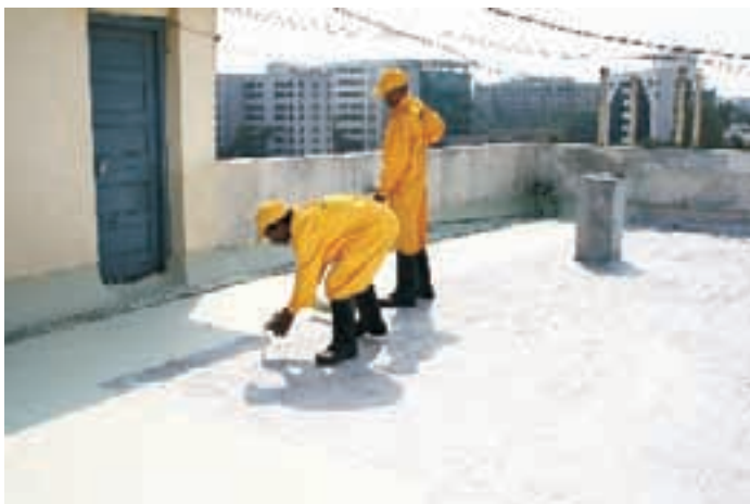
Spreading of material in pre-marked bays
