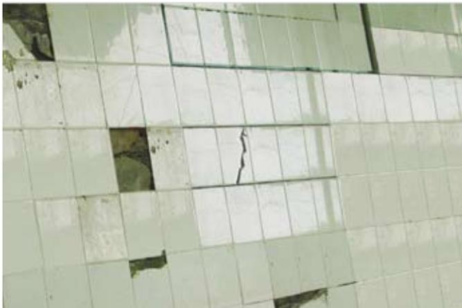
Fig 2 : Failure due to thermal movement
