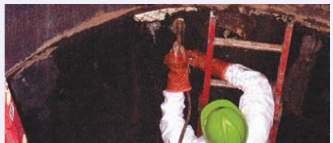
An injection specialist uses chemical grout to repair a leaking joint
