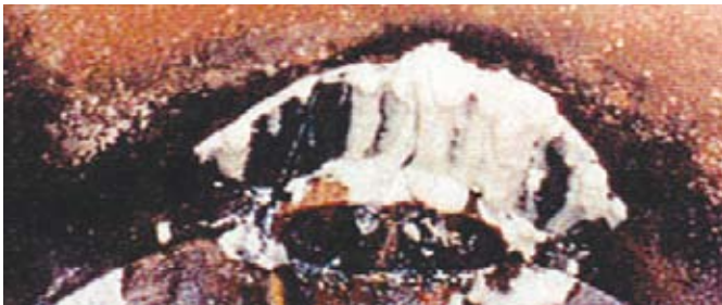
Hydrophilic chemical grout is injected around the area.
