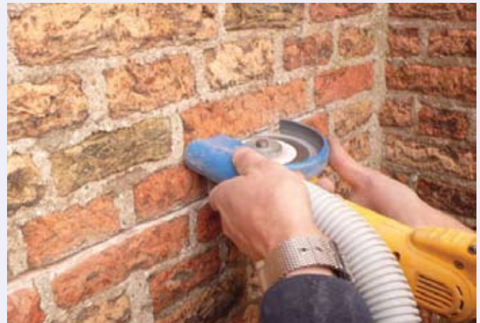
Fig: 6 Raking out of joints mechanically
