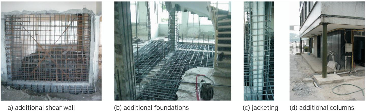
**Fig. 2** Applications of conventional strengthening methods
