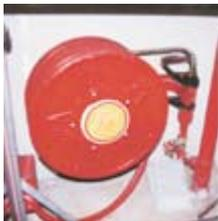
Fig. 5: Fire hydrant/hose reel
