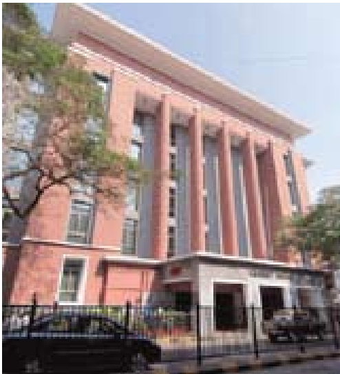
Fig. 1: Cement House (ACC) on Maharshi Karve road, Mumbai
