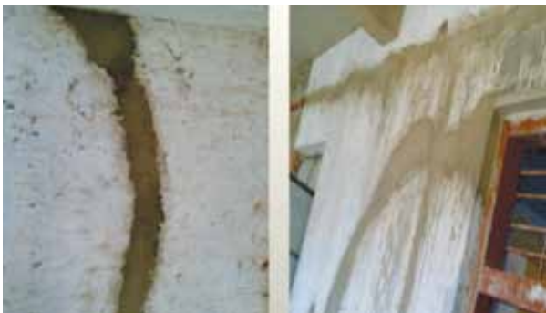
Fig. 7: Plastering cracks repaired
