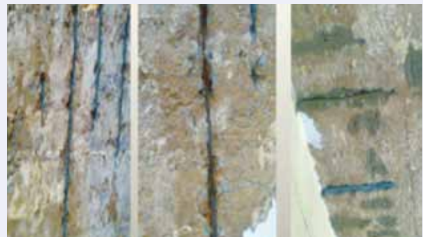
Fig. 9: Repairing of ceiling, beam
