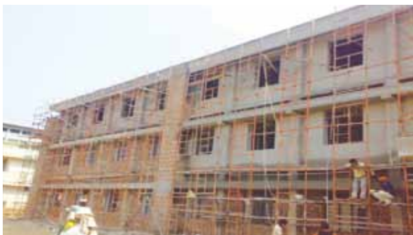
Fig. 11: Plaster finishes with polymer modified mortar
