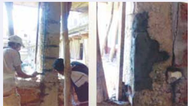
Fig. 8: Columns repaired with structural grade mortar
