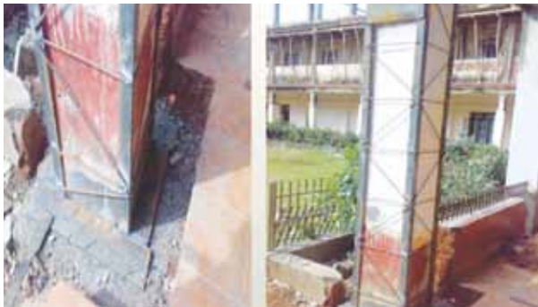
Fig. 10: Strengthening of columns by steel jacking
