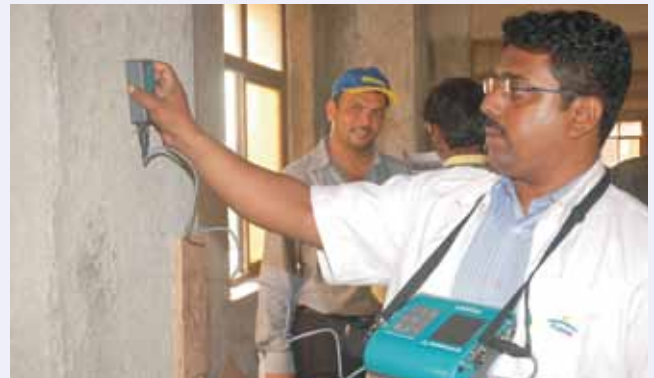
Fig. 1: Scanning of reinforcement by a Profometer
