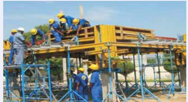
Fig. 2: Hands on training on Formwork and Shuttering in L&T (ECC) programme
