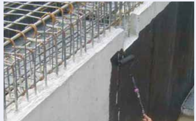
Fig. 8: Application of polymer-modified bituminous coating in a shallow basement
