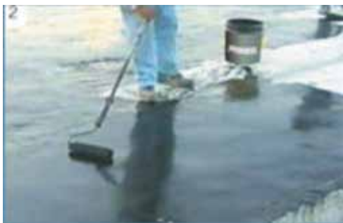
b. Apply primer coat with solvent based bitumen primer
