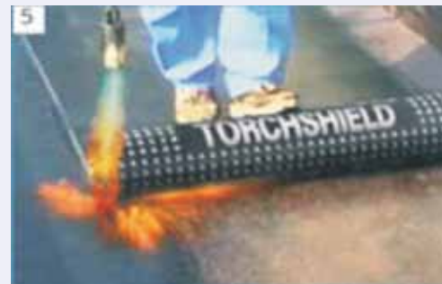
e. Use gas burner to heat substrate & underside to softening points
