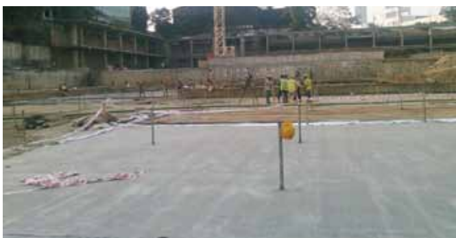
Fig. 13: View of EPDM based waterproofing membrane system
