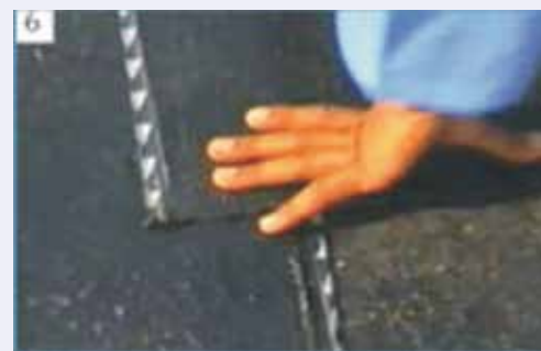
f. Keep overlap margin for minimum 100 mm
