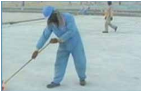
a. Clean & remove dust, dirt, loose particles and unsound substrate
