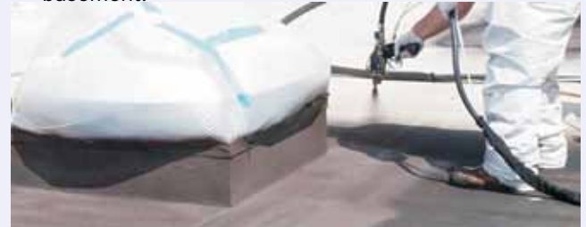
Fig. 14: Spraying of Hybrid Rubber Neoprene system
