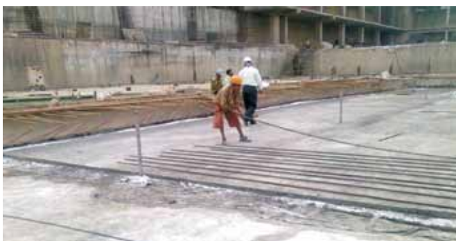
Fig. 12: Installation of EPDM based membrane system
