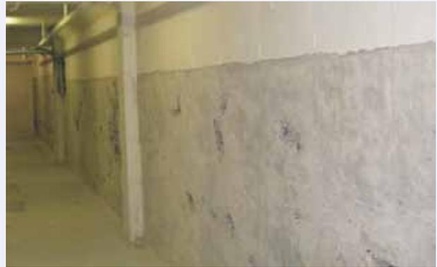
**Fig. 1:** Crystalline waterproofing on negative side
