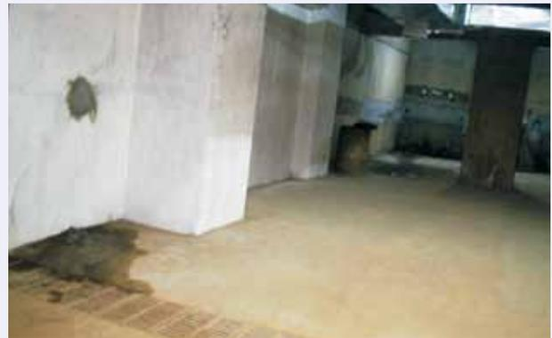
**Fig. 3:** Dampness and seepages in basement
