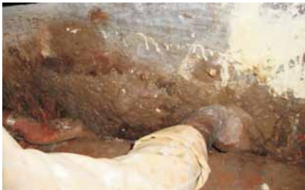
**Fig. 3:** Foam injection carried out in a deep basement wall
