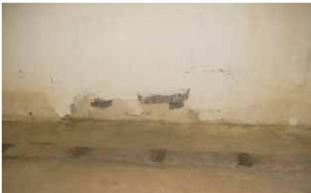
**Fig. 2:** Spalling of concrete due to corrosion in basement wall at floor level
