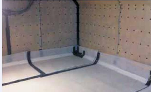
**Fig. 1:** View of cavity drain installation
