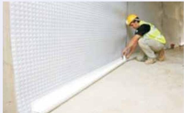
**Fig. 2:** Cavity mesh wall membrane curtain being hung down during installation
