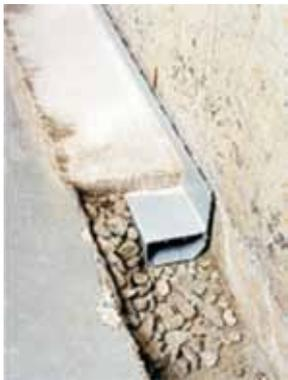
**Fig. 7:** Installation of footing drain pipe at wall and floor junction
