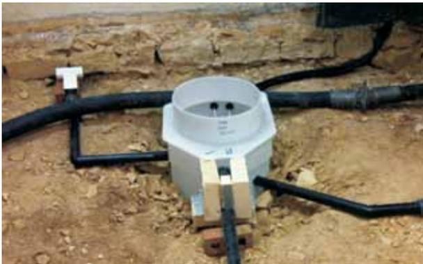
**Fig. 9:** Sump chamber for housing two medium duty Pumps
