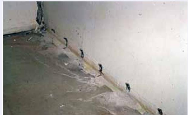
**Fig. 5:** Injection to basement wall at floor level for preventing rising dampness
