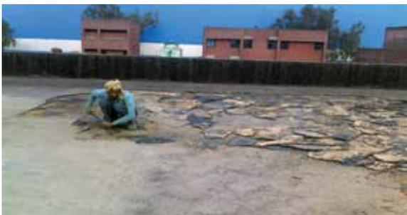
**Fig. 4:** Removal of existing waterproofing layer in progress
