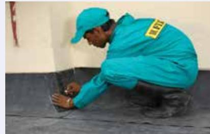
**Fig. 16k:** Marking on the membrane for splicing of cut piece at the corner junction
