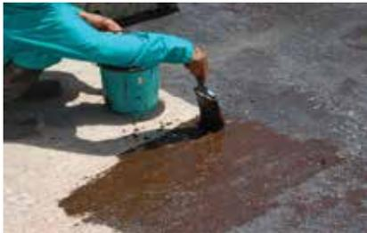
**Fig. 16d:** Application of bonding adhesive
