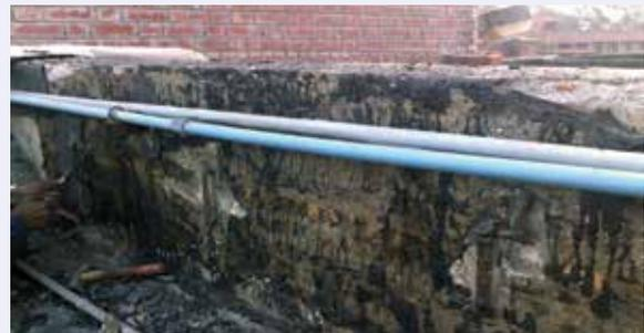
**Fig. 6:** Tar felting layer chipping off from parapet wall
