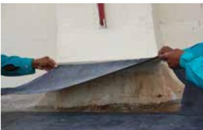
**Fig. 16i:** Aligning and laying the cut piece membrane
