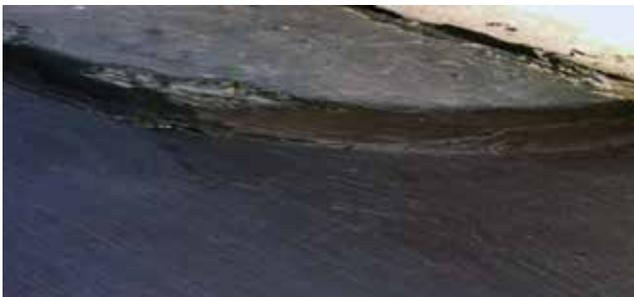
**Fig. 9:** First layer of bituminous coating
