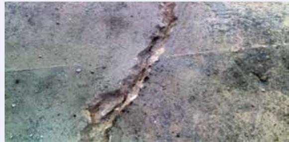
**Fig. 5:** Wider cracks on parent slab
