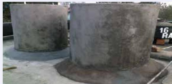
**Fig. 7:** After surface preparation and making watta at junction
