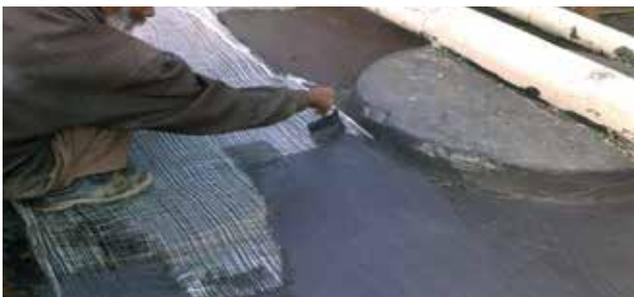
**Fig. 10:** Fibre mesh being sandwiched between first and second coat
