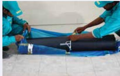
**Fig. 16e:** Opening the membrane from sealed cover
