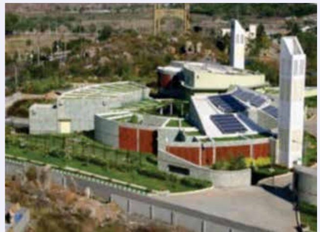
Fig. 2: Extensive green roofs, or roof gardens, cover 55% total roof surface area.
