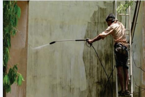
**Fig. 5:** Surface cleaning by water jetting
