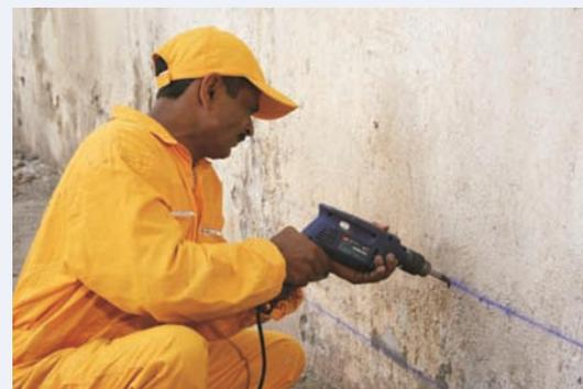
Fig. 3: Drilling holes for fixing nozzles for grouting
