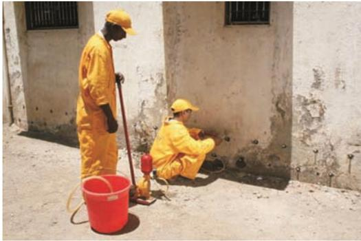
Fig. 2: Injection grouting for raising dampness
