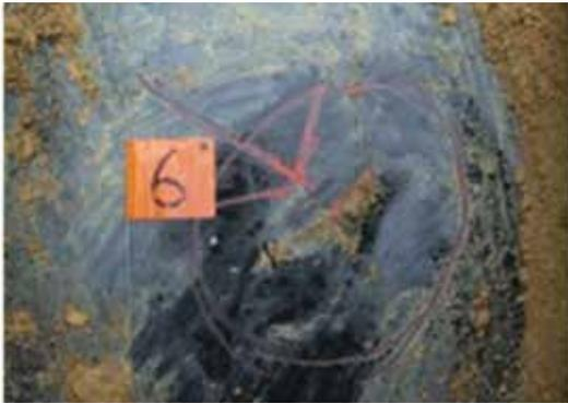
Fig. 9: Remedial waterproofing at leakage point
