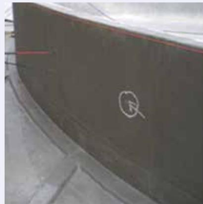
Fig. 12: Remedial waterproofing at leakage point
