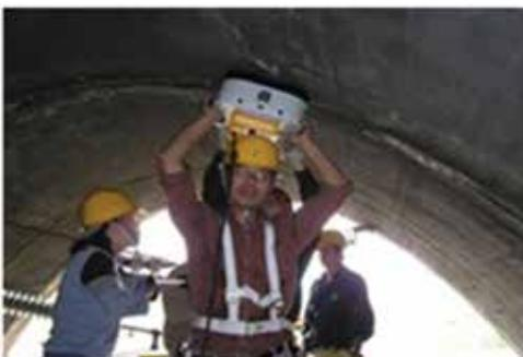
Fig. 5: GPR survey for detecting defects in a tunnel
