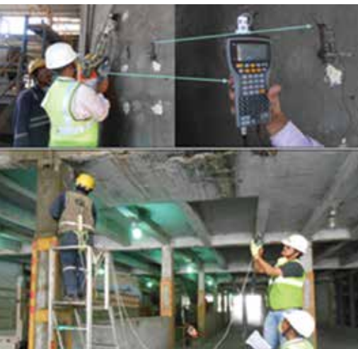
Corrosion investigation by Galvapulse GP 5000 in a cement plant
