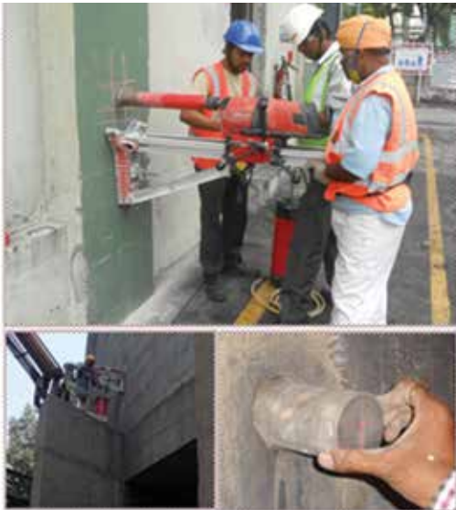
Structural audit of a cement plant
