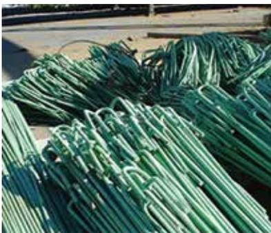
Fig. 2: Epoxy coated rebar for corrosion protection
