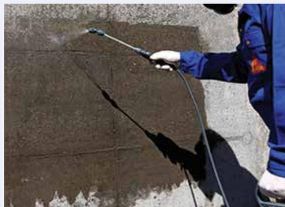
**Fig. 6:** Spray application for migration of corrosion inhibitors
