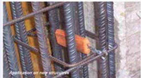
Fig. 3: Zinc casing in reinforcement as a sacrificial anode for corrosion protection
