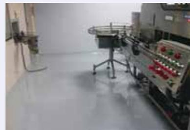
**Fig. 4:** Epoxy flooring in a Pharmaceutical laboratory
