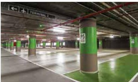
Fig. 7: View of polyurethane floor coating at parking in Terminal T2 of Mumbai International Airport
