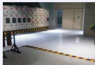
**Fig. 5:** Epoxy flooring in an Electrical Panel board room for antistatic properties
