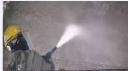
Fig. 8: Sand blasting for concrete removal
