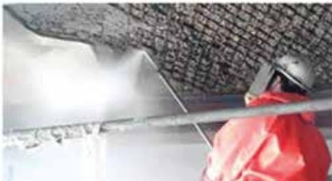
Fig. 7: Hydrodemolition for concrete removal
