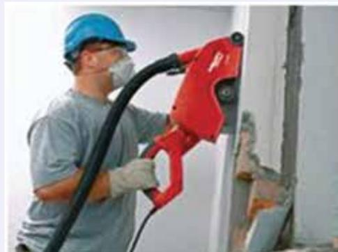
Fig. 3: Hand held saw cutting of column surface
