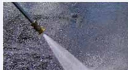
Fig. 12: VHigh-pressure water blasting for concrete cleaning
