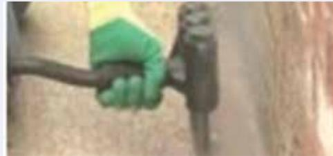
Fig. 5: View of scabblers for concrete removal
