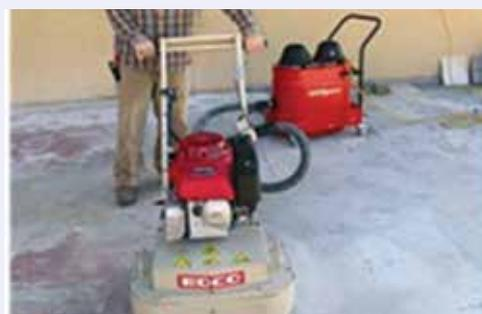
Fig. 6: Concrete scarifier during surface cutting
