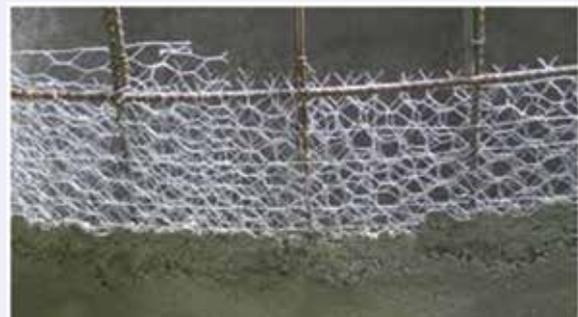
**Fig. 9:** View of ferrocement repair of concrete with welded wire mesh reinforcement
