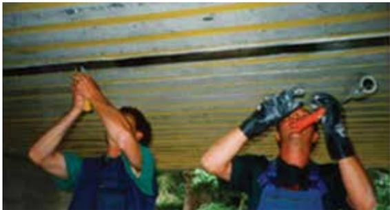
**Fig. 3:** A roof slab being strengthened with FRP strips
