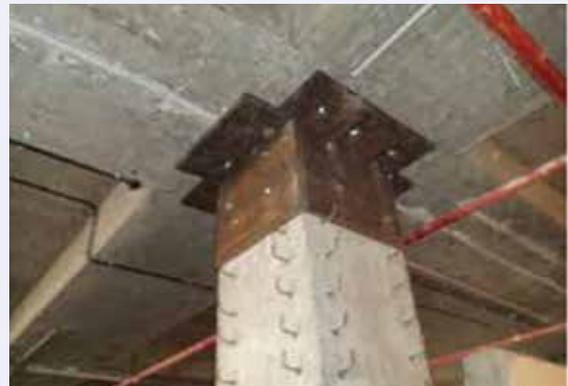
**Fig. 6:** A column being strengthened with steel plate bonding
