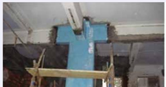
Fig. 2: A column being strengthened with FRP sheets
