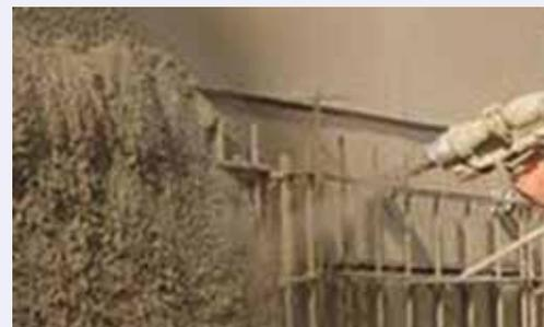
Fig. 10: View of concrete repair by shotcrete method
