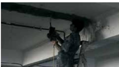
Fig. 2 e: Injection in underside
