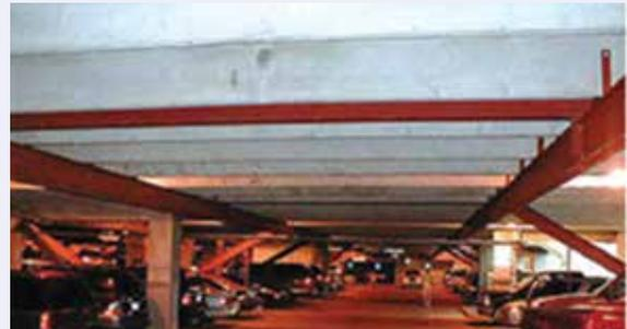
Fig. 1: View of span shortening by providing structural steel members in a parking deck
