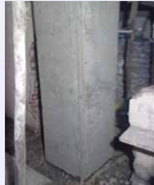
Fig. 7: Column after micro concreting
