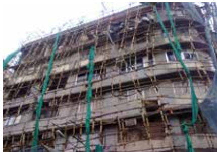
Fig. 1: Continuous sunshade being provided
