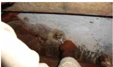
Fig. 5: Screwing of packers tightly.
