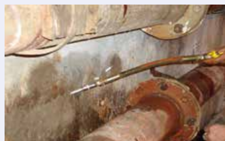
Fig. 7: PU Injection in process
