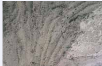
Fig. 9: Finishing of spalled repair
