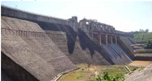
Fig. 1: A panoramic view of Muran Dam.
