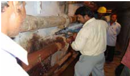
Fig. 3. Drilling holes with drill machine
