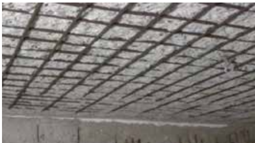
Fig. 4: Roof slab before micro concreting
