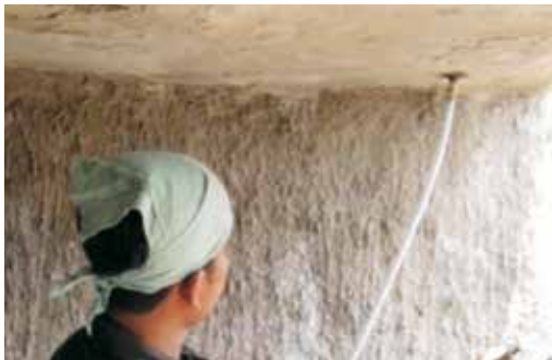
Fig. 12: Epoxy injection through nozzle
