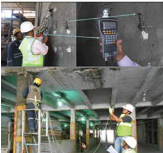
Corrosion investigation by Galvapulse GP 5000 in a cement plant
