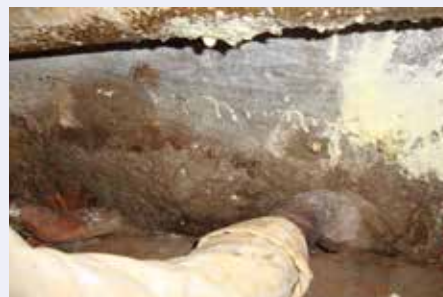
Fig. 9: Filling the drill holes with polymeric grout.
