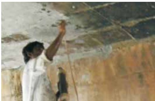
Fig. 13: Epoxy injection in progress at different location
