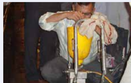
Fig. 6: Pumping being ready after mixing of materials
