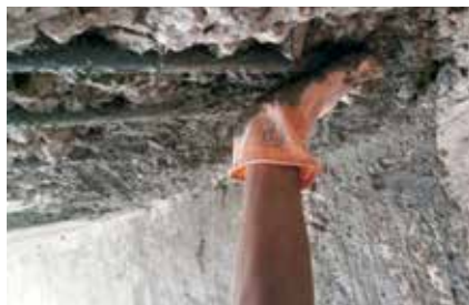
Fig. 7: Applying structural grade mortar
