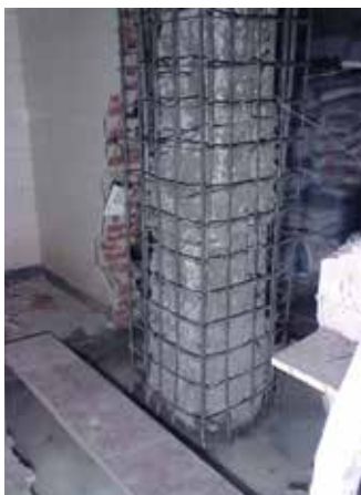
Fig. 6: Column before micro concreting
