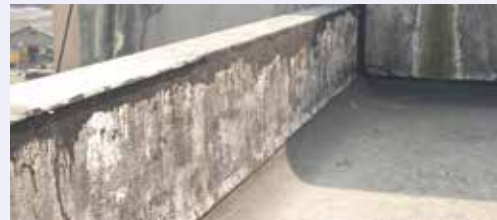
Fig. 2: RCC coping before
