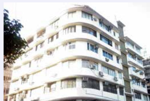
Fig. 9: View after repair
