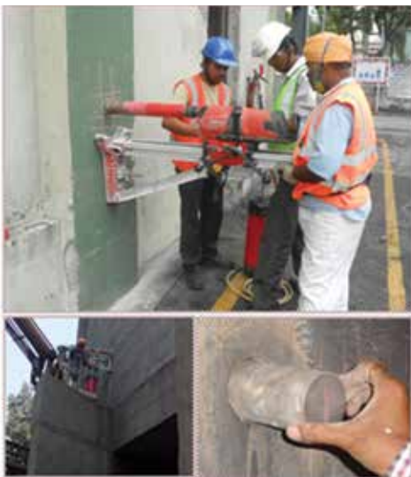
Structural audit of a cement plant
