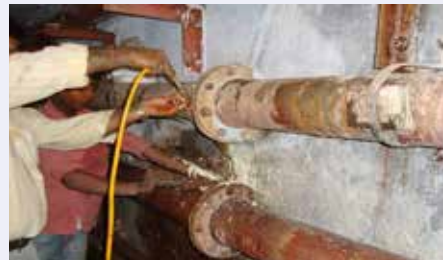
Fig. 8: Continuing with secondary PU Injection
