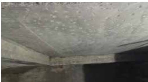
Fig. 5: Roof slab after micro concreting
