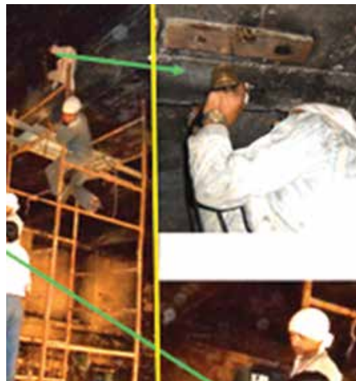
Fire damage assessment of an auditorium building
