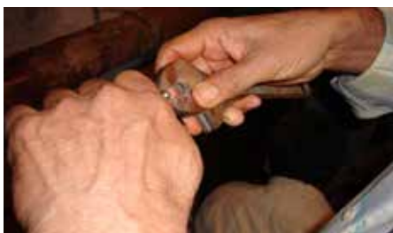
Fig. 4. Instalation of packers in the holes.
