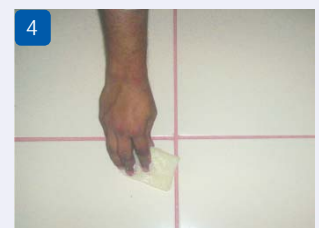
4 Clean the grouted joints with damp sponge diagonally
