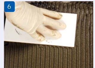
6 Start placing the tiles with slight twisting action
