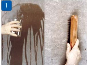
1 Clean the tiling substrate thoroughly
