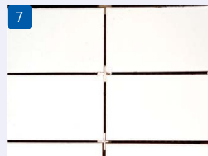
7 Continue tiling by keeping at least 2mm joints between tiles
