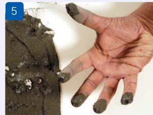
5 Touch the paste intermittently and if sticks to finger then continue tiling
