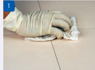
1 Clean existing tiles thoroughly. Mild acid etching followed by water washing is preferred
