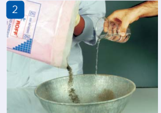
2 Mix powder to water/liquid in proportion 2.5 to 1 part by volume
