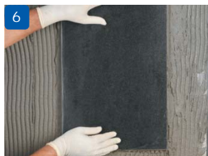
6 Start placing stone tiles
