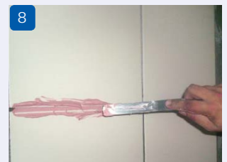
8 Start filling joints by pressing paste firmly
