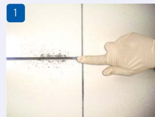
1 Clean the tiling substrate thoroughly
