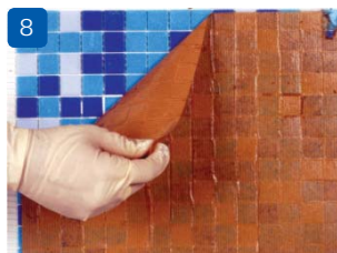
8 Remove the backing paper after 24 hrs & clean the tiles
