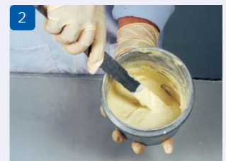
2 Mix it thoroughly until a homogeneous paste is obtained
