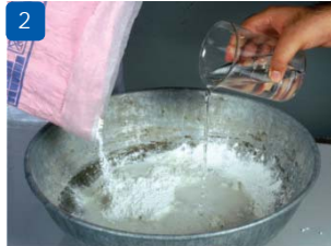
2 Mix powder to water in proportion 2.5 part to 1 part by volume
