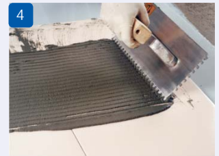
4 Apply the paste on existing tiles with 3 or 6 mm notch trowel
