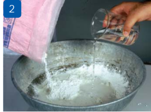
2 Mix powder to water in proportion 3 part to 1 part by volume
