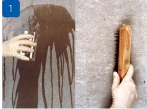
1 Clean the tiling substrate thoroughly
