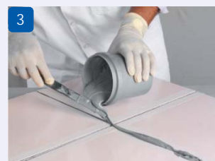
3 Start filling joints by pressing paste firmly
