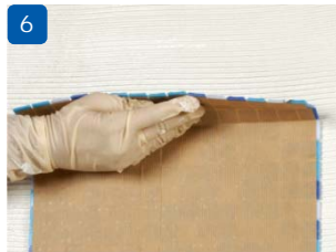
6 Start placing glass mosaic sheets with slight twisting action
