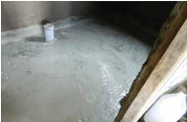
Fig. 28: Screeding after waterproofing
