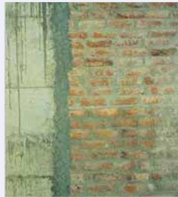
**Fig. 7:** Reinforcement installed at brick - RC joint
