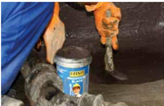
**Fig. 17:** Bituminous elastomeric coating in sunken floor of a bath room
