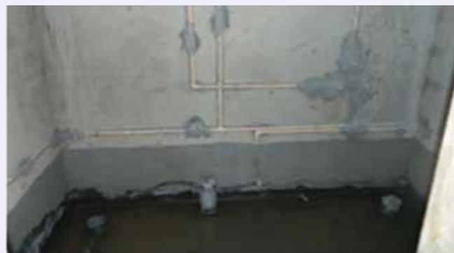
Fig. 27: Water ponding test after waterproofing in bath room
