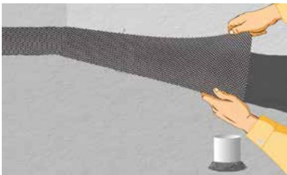
Fig. 21: Laying of glass fibre mesh
